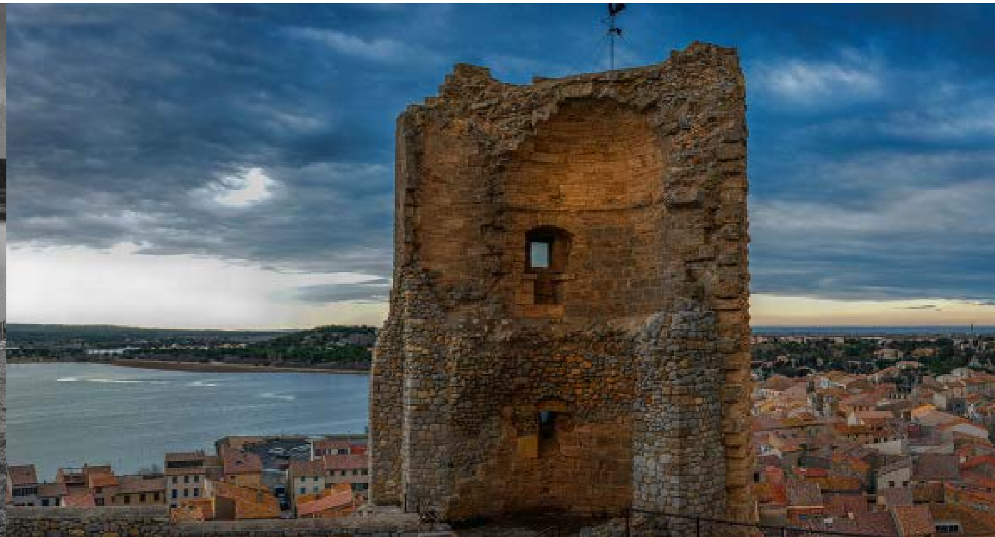
OPPOSITE: The 13th century, medieval Caerphilly Castle, Wales, UK. It is the second largest castle in Britain, and is memorable for having introduced concentric castle defence design to Britain. ABOVE: The ruins of the 10th century Tour Barberousse (Redbeard Tower) of Gruissan castle, Occitanie, France. The castle was designed to observe the approaches to the harbour at Narbonne and to guard against seaborne invasions of the city.
